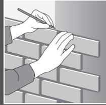
**B.** From this line, mark a parallel line away from the wall at a distance equal to double the thickness of the panel - between 2 and 4 cm depending on the model. (This will be the outside line of the cut)
